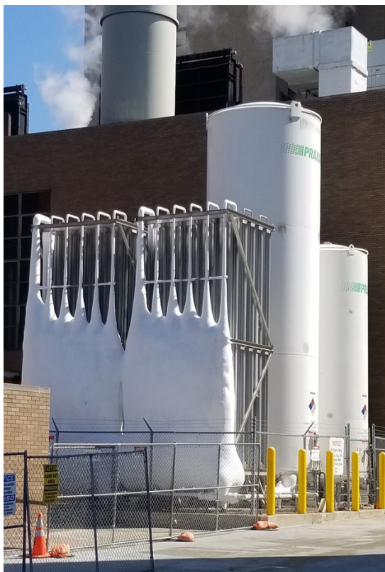
Typical hospital liquid oxygen system including two main reservoirs and a smaller reserve reservoir. The vaporizing coils are in the foreground.
