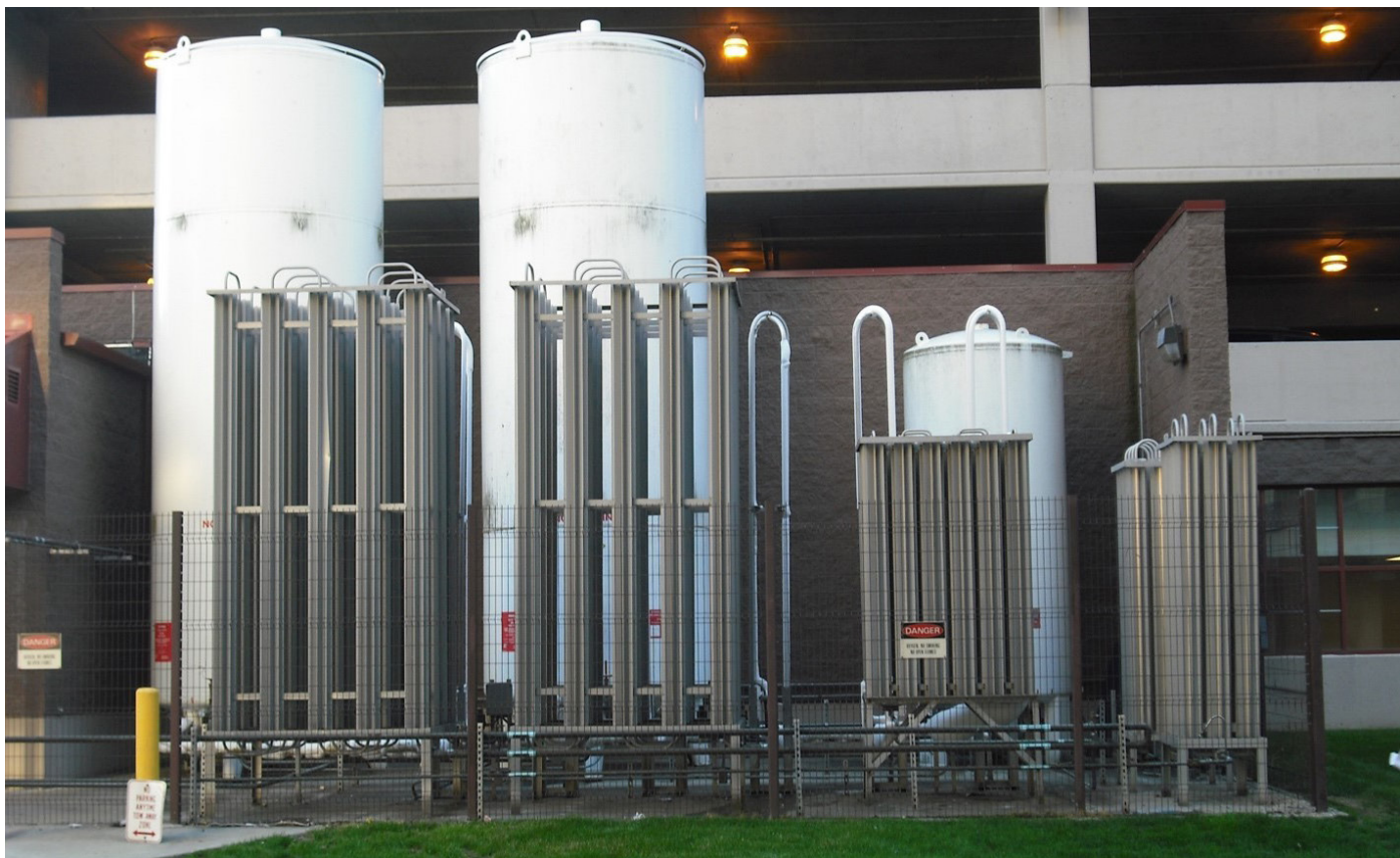
Typical hospital liquid oxygen system including two main reservoirs and a smaller reserve reservoir. The vaporizing coils are in the foreground.
